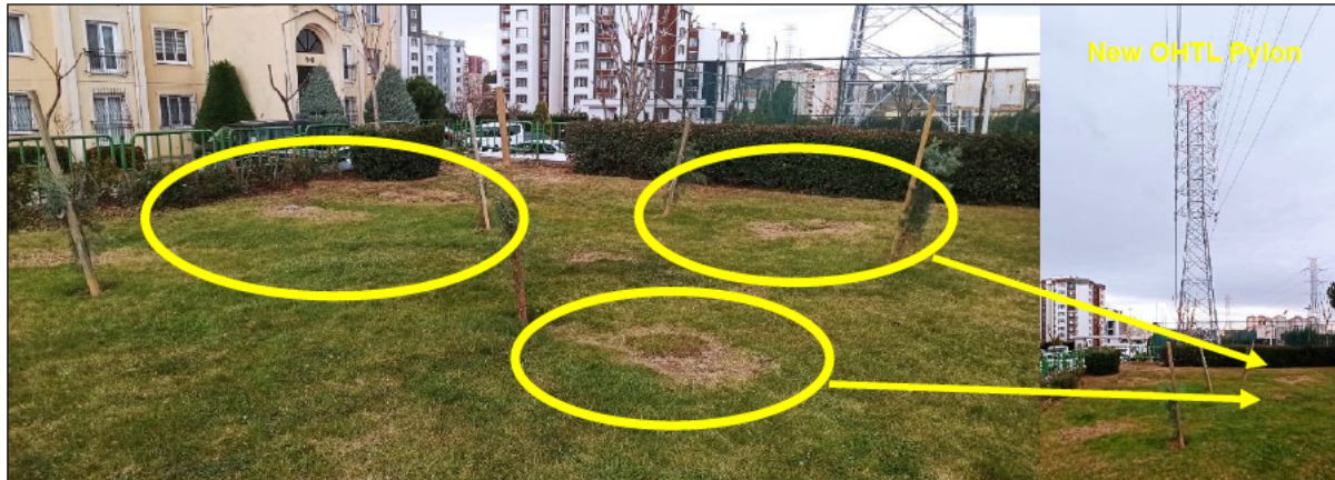
Figure 2-26. Rehabilitated OHTL Pylon Locations on Previous Route and the New OHTL Pylon Built on Private Parcels
